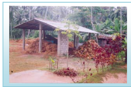
Coir processing Centre and the Machinery
